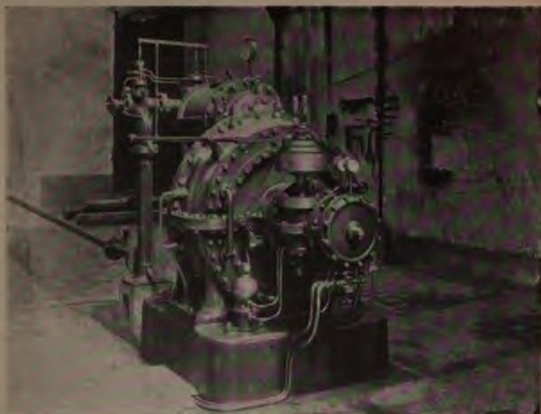
FIG. 82.—The Armengaud and Lemale gas turbine. A view of the 500 horse-power turbine in the experimental laboratory at St. Denis.
